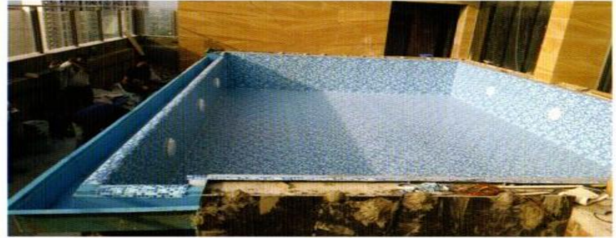
2. Pasting of Liner and Under water lights along with other fixtures.
