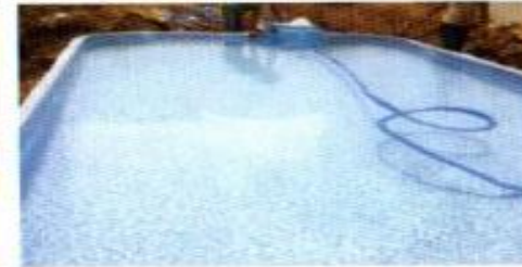
Prefab Pool at GHANDI NAGAR GUJARAT
