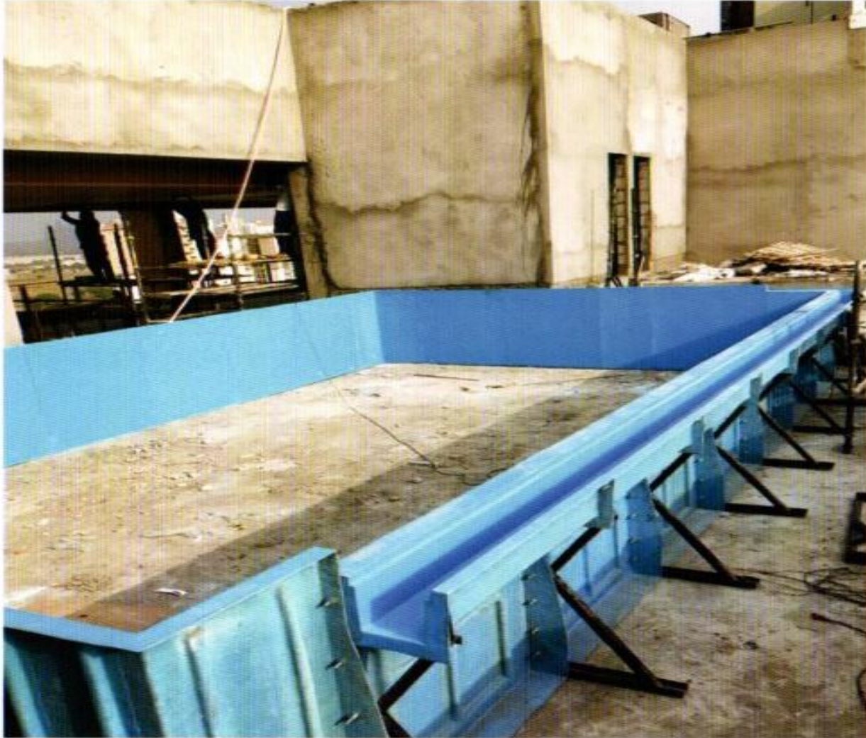
1. Step : Panels erecting
