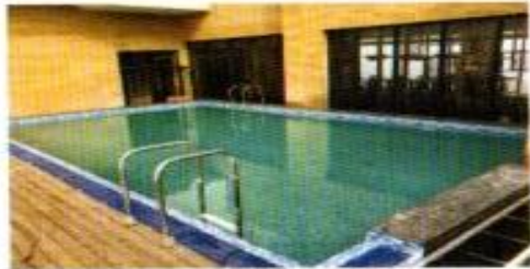
Overflow Prefab Swimming Pool at HOLIDAY INN
